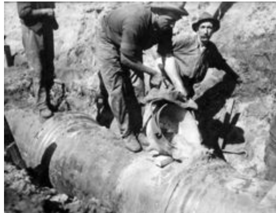
Pouring molten lead 1925. Courtesy: Western Power.
