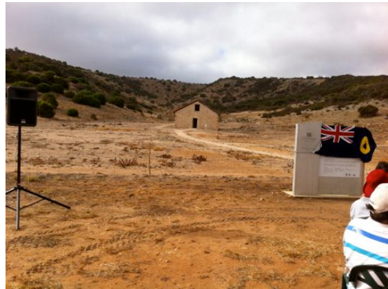
Restored Convict Depot. First completed in 1855. Photograph taken 26 January 2014 by J. Weir.
